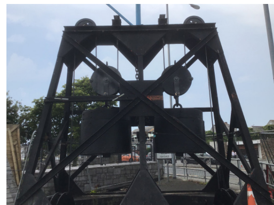
New gantry sheave re-installed
