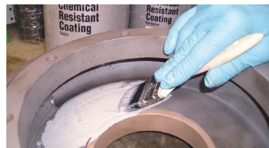
Applying wear resistant coatings to the internal components
