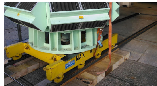
Pump and motor loaded onto bespoke track system
