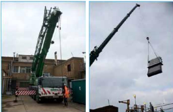
ERIKS completed a site survey and provided the customer with a detailed plant & site survey for each screen to accompany each quotation. Once ERIKS recieved the go ahead for the project the removal and transportation of the screens to the dedicated screen workshop was completed using fully insured Contract Lifts to comply with regulations.
