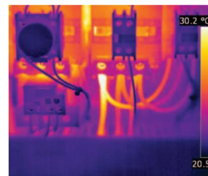
The customer took no action on the thermal exception, believing 30.2°C was not an issue. However, using the ERIKS severity calculation, a defect of 250% is revealed!
